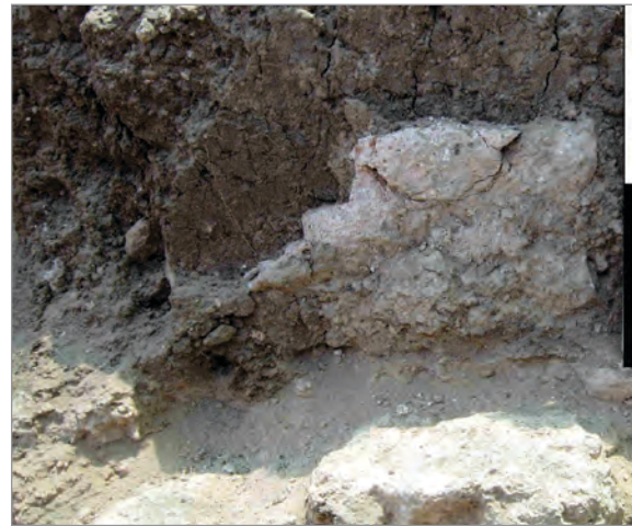
Figure 6. Area A: Plaster remains over the aqueduct's fill in the area where the northern wall was removed.
