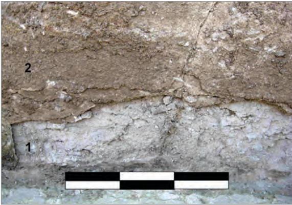
Figure 7. Area A: The two layers of plaster from the section where the northern wall was removed, earlier layer (1) and later layer (2).
