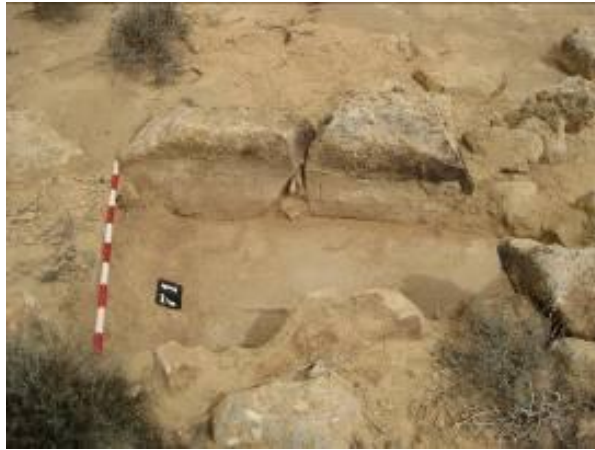
Figure 17: The dam's eastern courses resting on bedrock.
