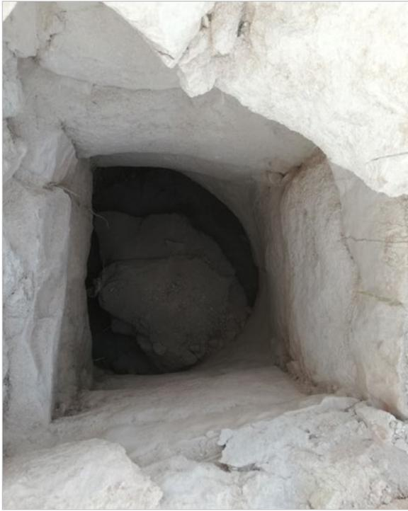
**Figure 10.** The opening of the cistern hewn into the *nari*.
