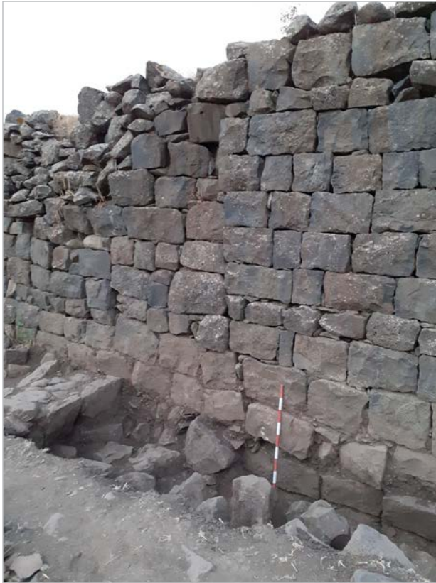
Figure 5.32. The seam between the two units along the northern façade of the standing Hauranian house.
