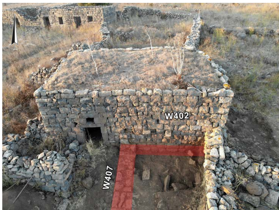
Figure 6.41. The Byzantine walls of the Area NH house, marked in red, incorporated into the 20th century house (Photo by Dan Malkinson).
