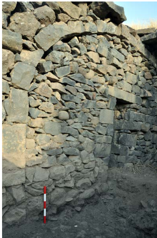
Figure 5.39. A filled arch in the southern wing.
