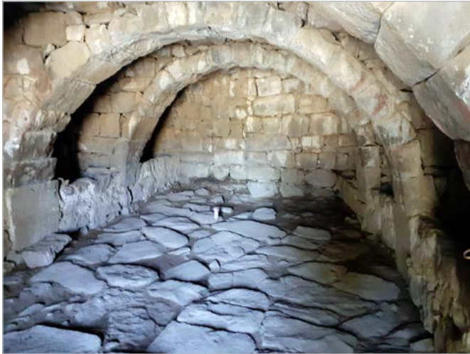
Figure 5.30. Hall of Arches in the standing Hauranian house, looking south. Note the troughs between the arches (photograph by Shai Scharfberg).
