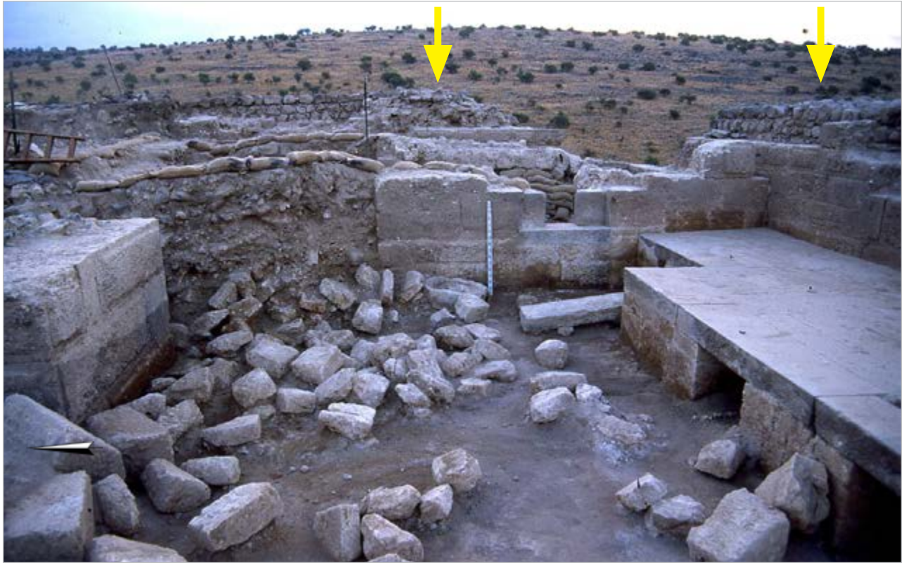
Figure 4.7. Remains of the collapsed vault on the kitchen floor in Area E, looking east. Note the ashlar casing and basalt core (marked with yellow arrows).
