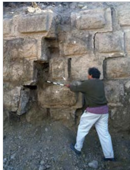
Figure 18.5. Ronnie Ellenblum with a 50 cm scale bar right after the excavation of the faulted northern wall, in 1994.
