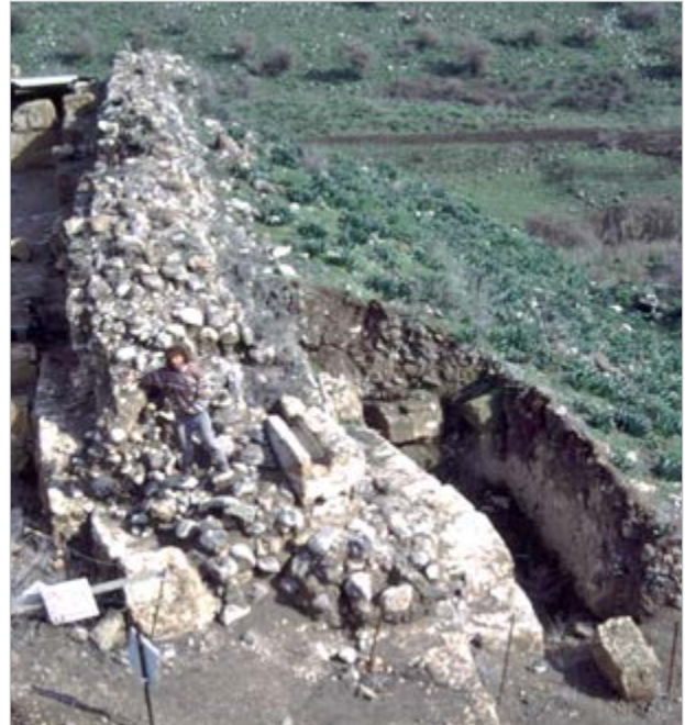
Figure 18.3. Looking east, displacement of the Frankish walls of Vadum Iacob in Area E.
