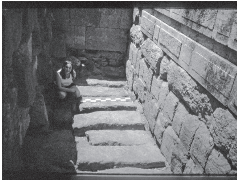
Figure 22.8. The ashlar-built platform (Bamah B) below the Hellenistic platform, Area T. Note the use of the headers-and-stretchers building technique. Drawing by Noga Zeevi.
